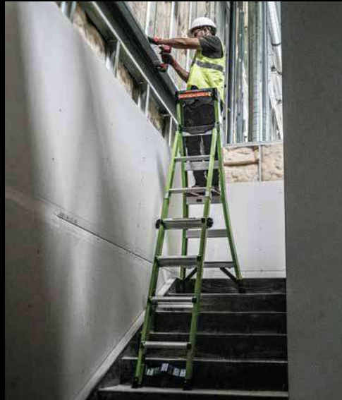
Extended Rear Section for Work on Stairs
